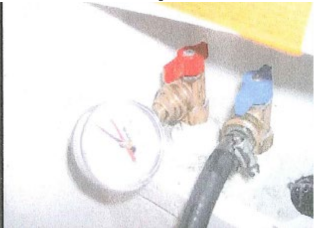
Pressure Testing both Hot & Cold Lines
