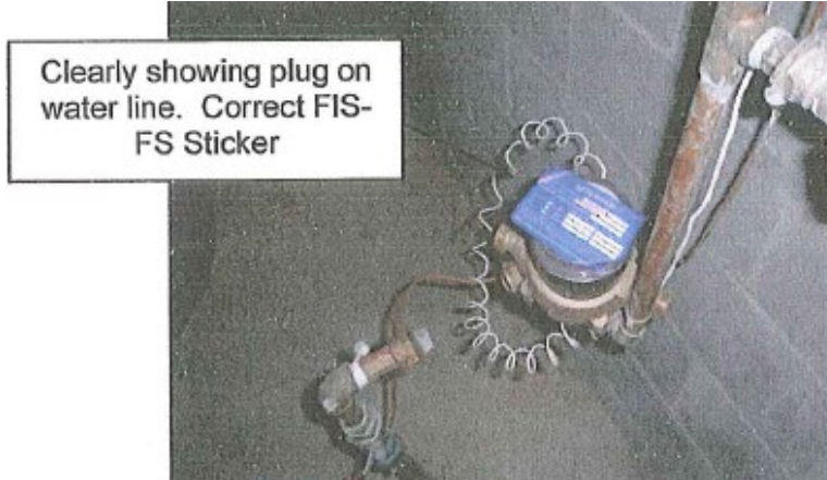
After water meter dropped & water line capped
