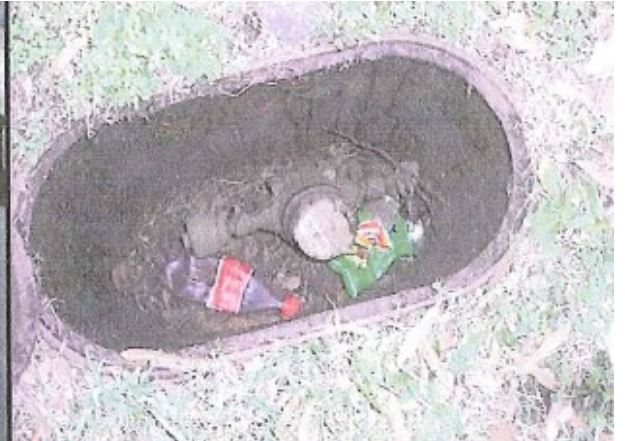
Water Meter on Exterior of Property
