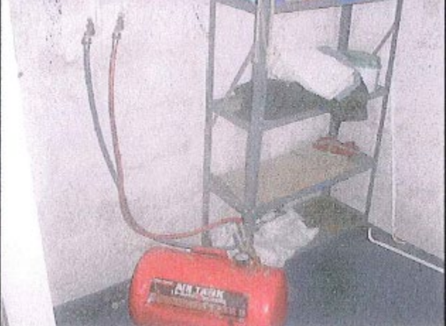
Pressure Testing Both Hot & Cold Lines
