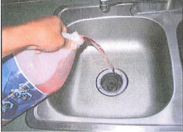
Adding Anti-Freeze to All Traps & Fixtures
