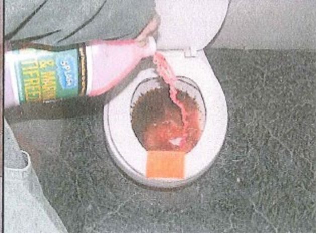
Incorrectly Winterizing a Dirty Commode
