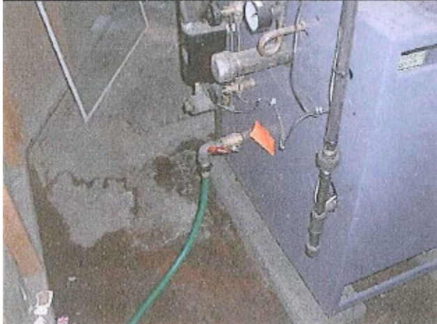
Draining of Boiler During Wet Winterization
